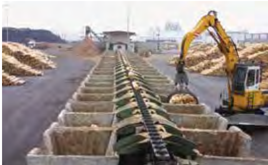
Sorting line/ bloch transport line
