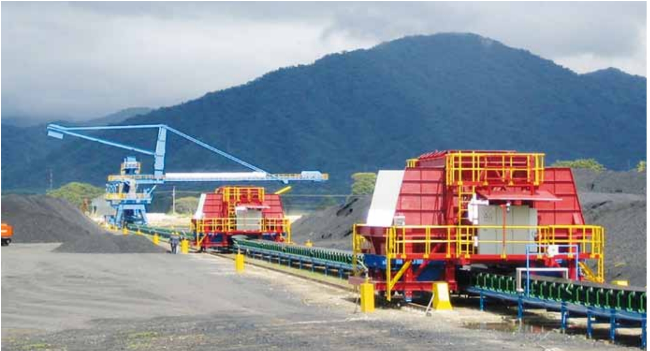
mineral deposits conveyor
