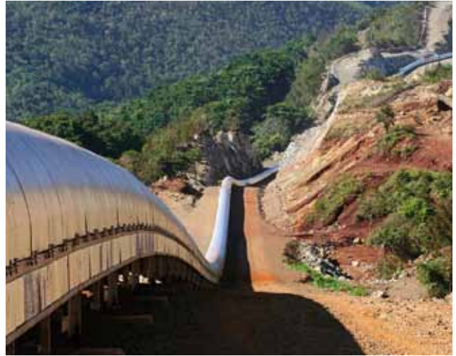
long distance conveyor
